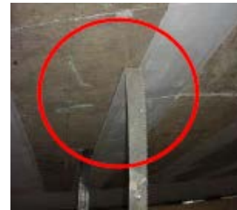
Epoxy bonding interface problem
