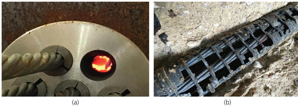
Figure 14. Fire damage of (a) PS tendon and (b) sheath tube
